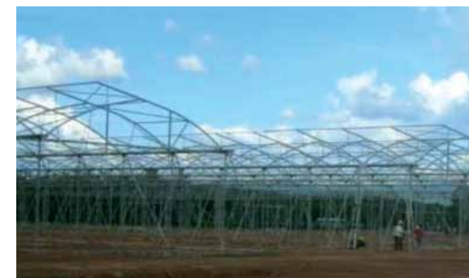
Greenhouse under construction in Bukit Kura, Kedah
