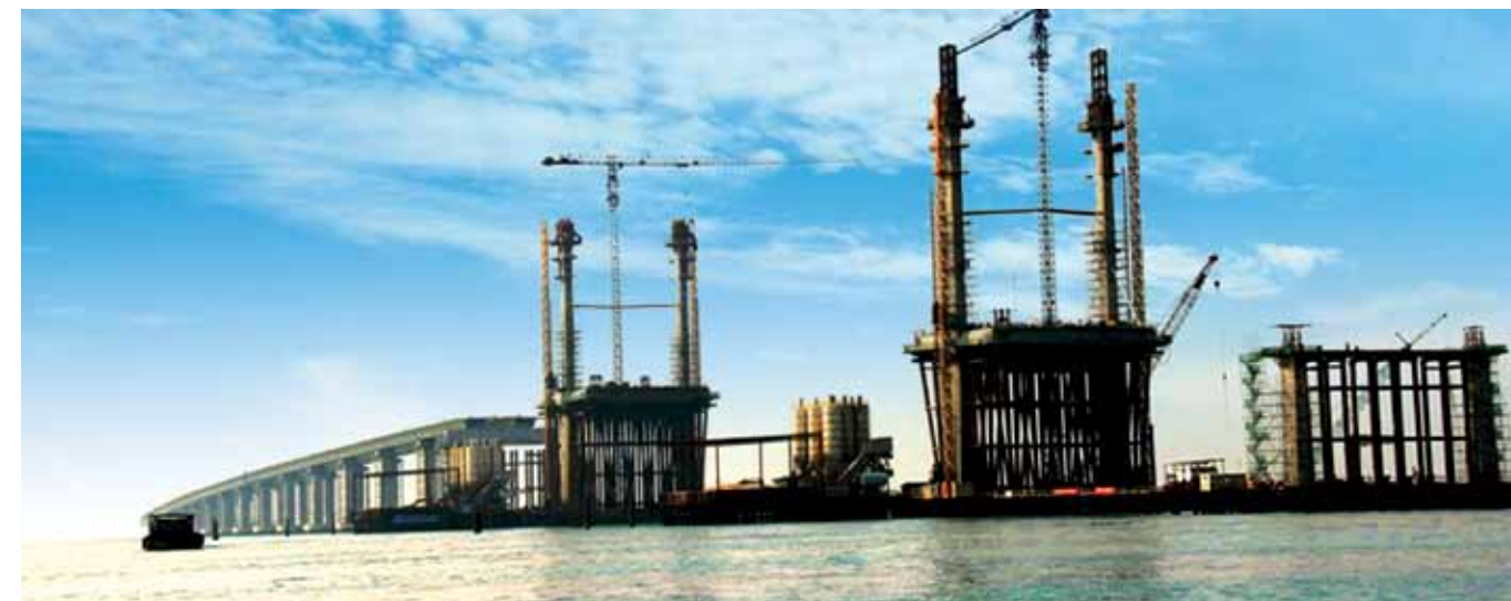
Construction of 2nd Penang Bridge well underway
