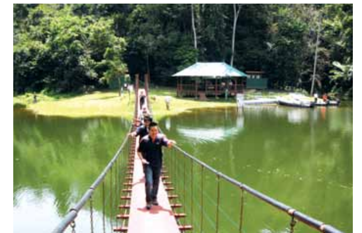
Existing base camp site, Sungai Papan, BTTR
