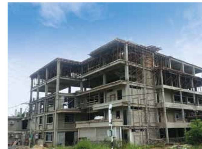
Construction of Zinon Food Industry's factory
