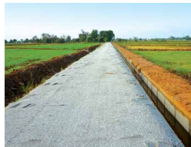
Infrastructure improvement on the road and drainage system
